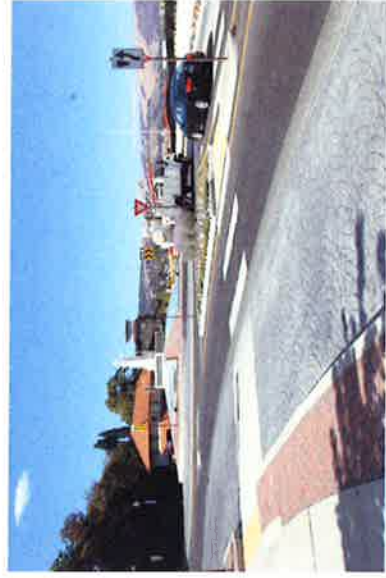
Below: a decorative modern roundabout in the town of The Dalles, Oregon, is a gateway into town and smoothly and safely handles even truck traffic, featuring a 3" tall truck "apron" around the outside edge of the roundabout that the largest trucks and emergency vehicles can use to drive over while turning, and there is even a decorative truck apron on the approaching street (bottom of image).
