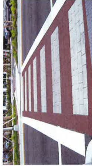
Above: This crossing includes bold ladder-style paint, colored pavers, and a "Z" crossing in the median, so that pedestrians are facing oncoming traffic before stepping into the street.
